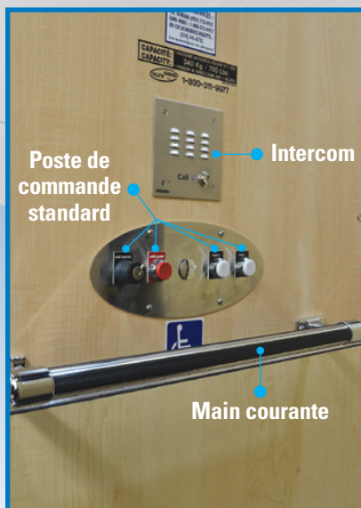
STATION DE COMMANDE
